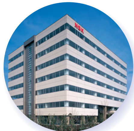
Bearing Technology Center (Japan)
